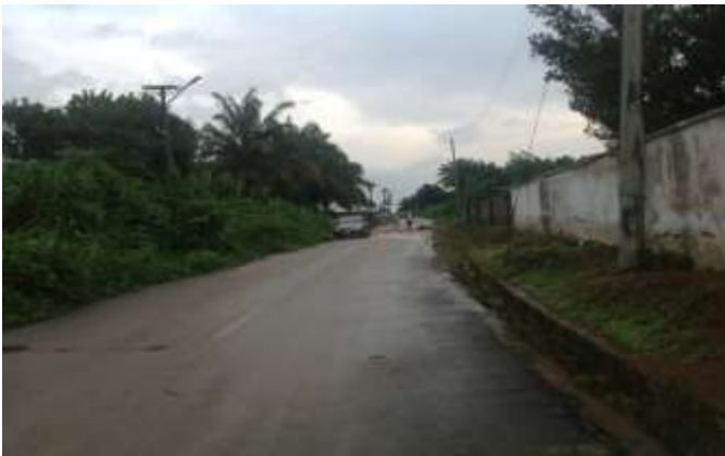
Plate 5: Showing the view of Makanjuola Road with drainage
