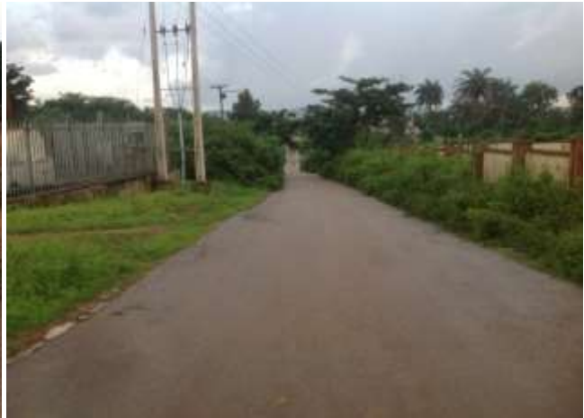
Plate 4: Showing the view of Okesina Road surface with little defects along road
