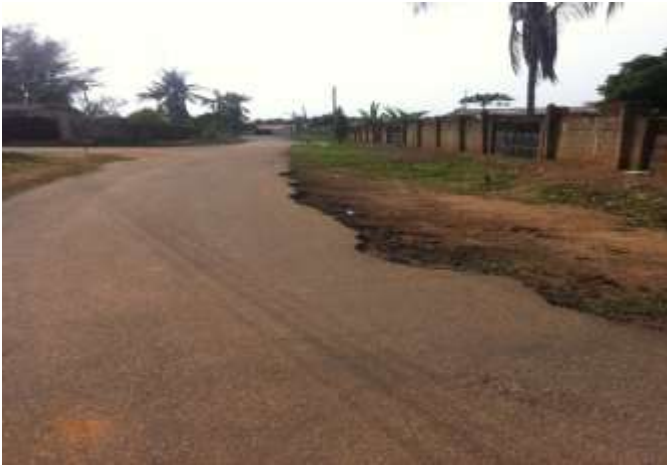
Plate 3: Showing the view of Cedars Road with edge cracks along the road
