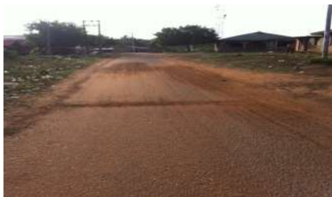
Plate 6: Showing the view of Iyalaje Road with surface defect
