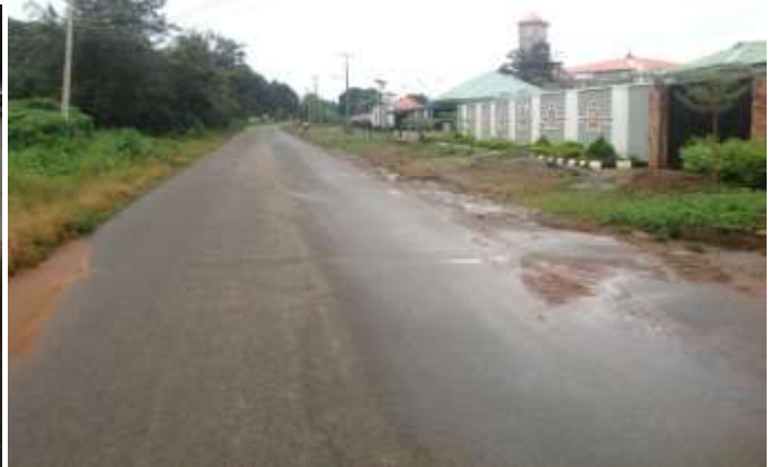
Plate 6: Showing the view of Igbaye Road with no drainage
