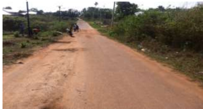
Plate 2: Showing the view of Olopade Oyinlola road with potholes
