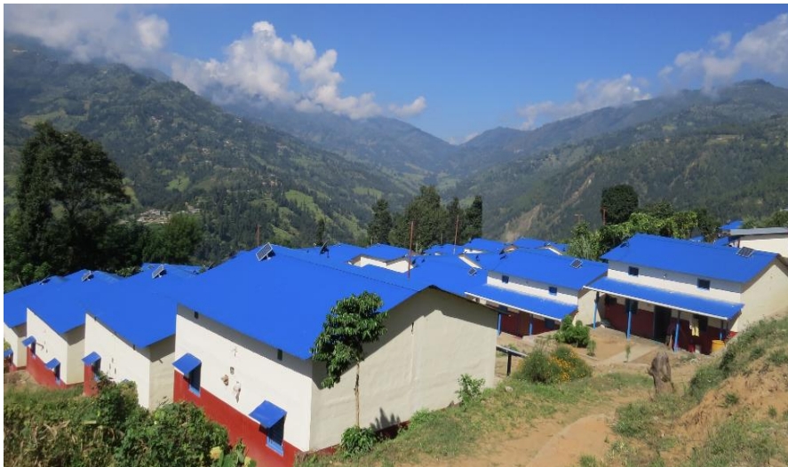
FIGURE 3. Completed houses of unified Giranchaur model village1
