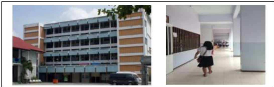
FIGURE 2. Showed the school buildings of Wat Nak Prok School in Pasri Chareon District
