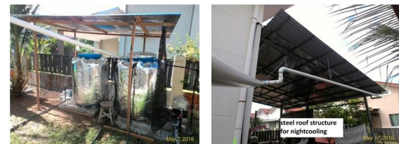
(a) 2 units of 200 gallon insulated water storage tanks with pump set (b) Pitch steel roof structure acting as a heat exchanger to cool water at night time
