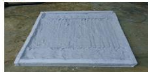
(c) Tubing fully embedded in screed layer.
